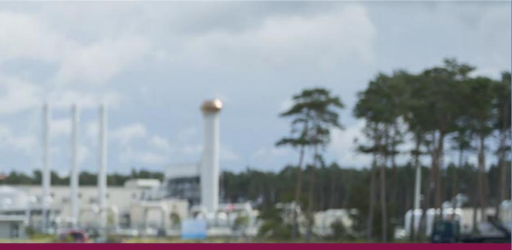
The station comprises two sections: an offshore section for the incoming Baltic Sea pipeline and an onshore section where the two downstream pipelines OPAL and NEL are located. The onshore section is divided into a 180 bar and a 105 bar section. The 180 bar area has filters, pre-heaters, and control valves. Mainly measuring and control systems operate in the 105 bar area.
