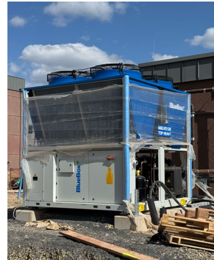
Multi-functional heat pump, Reckrod 2
